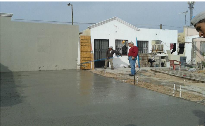
Pouring the cement slab in front
