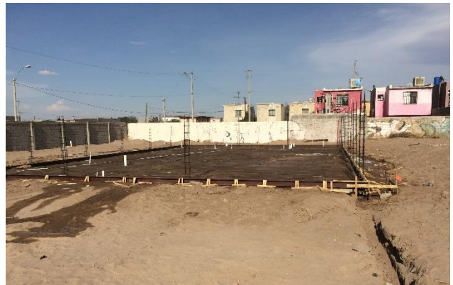
Plumbing in & Ready for Concrete
